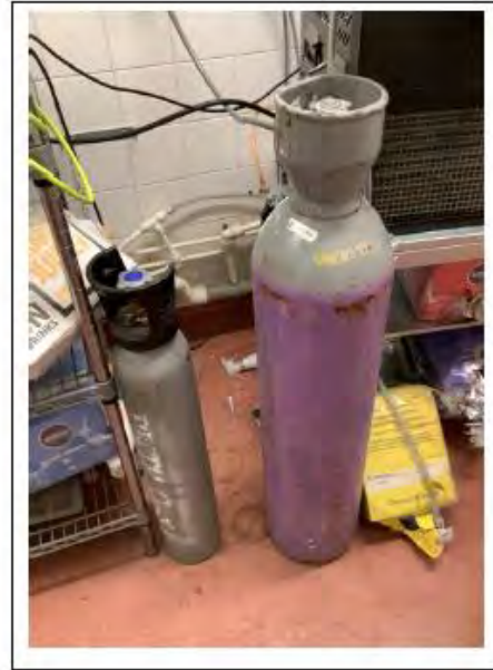
Example of the numerous unsecured gas cylinders
