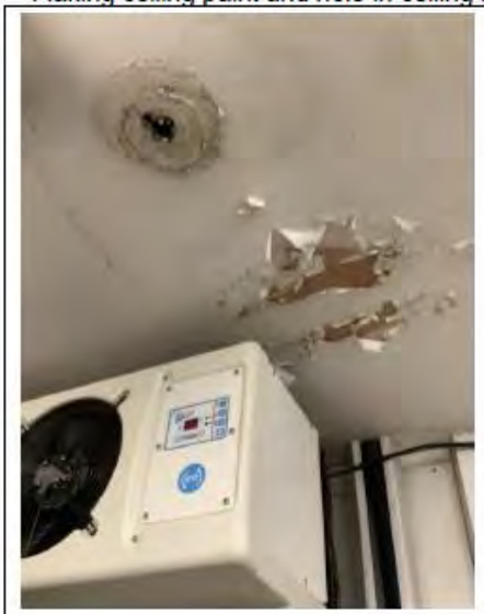
Flaking ceiling paint and hole in ceiling in cellar
